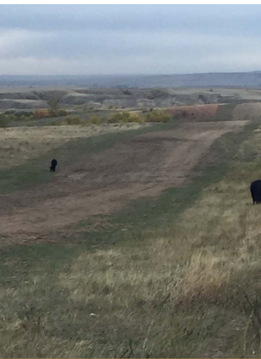
Unsuccessful reclamation of a grass seeding following pipeline installation. (NDSU photo)
