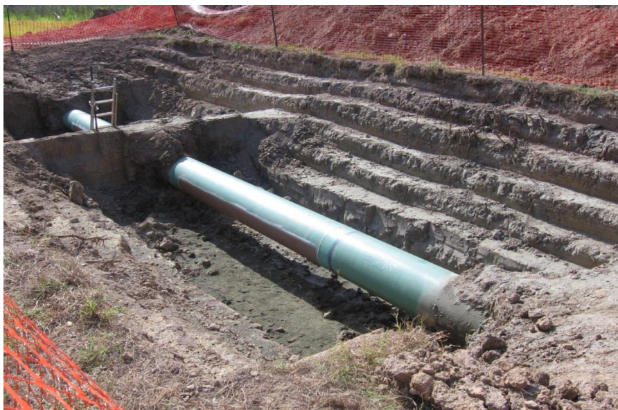
Confirmation Dig of Identified Pipe Joint
